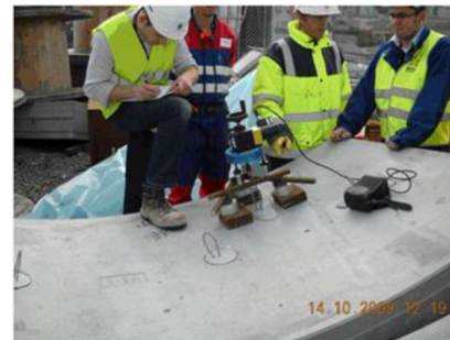
Figure 42: Smooth finish of a typical moulded tunnel lining segment.
