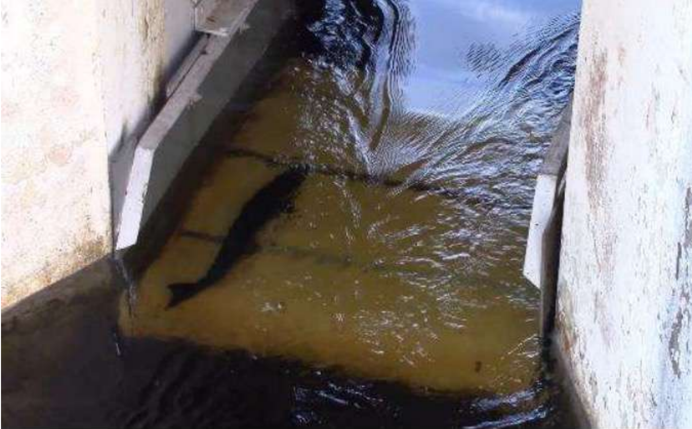
A salmon passing through the counting flume in a Borland fish lift
