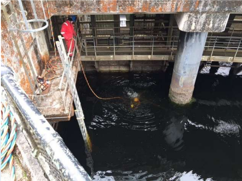
Diver installing study equipment
