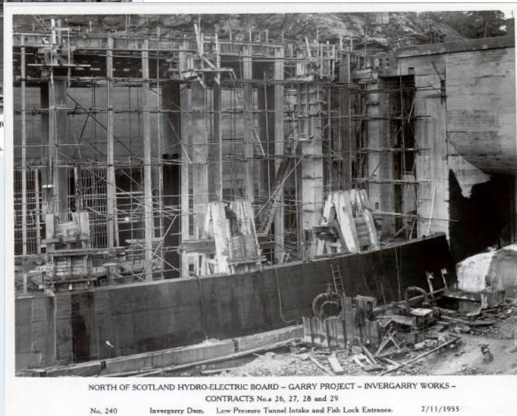
Photos of construction of Invergarry HEP station in 1955
