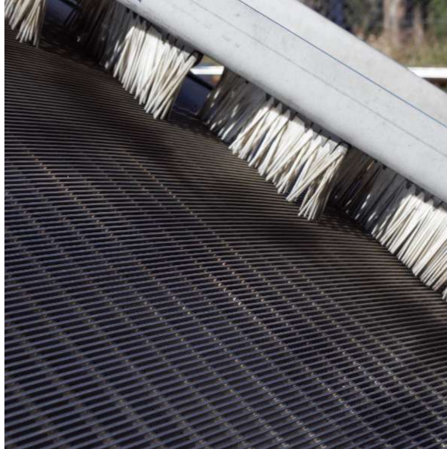
Performance of Australia's first brushed conical fish protection screen at a large irrigation pump diversion
