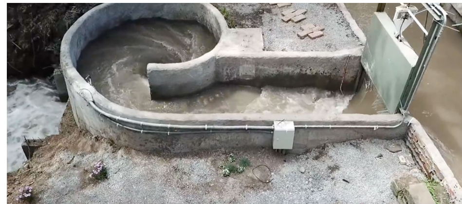
Hydropower generator Innovation > Science > Whirlpool turbine creates fish-friendly hydropower
