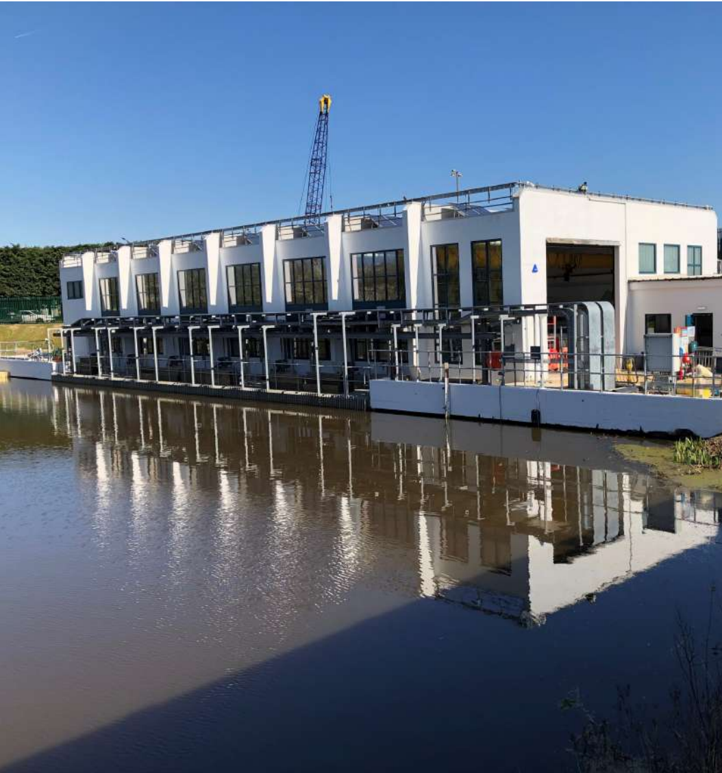
Keadby PS – 24m 3 /s capacity (6No 4m 3 /sec 330kW pumps)
