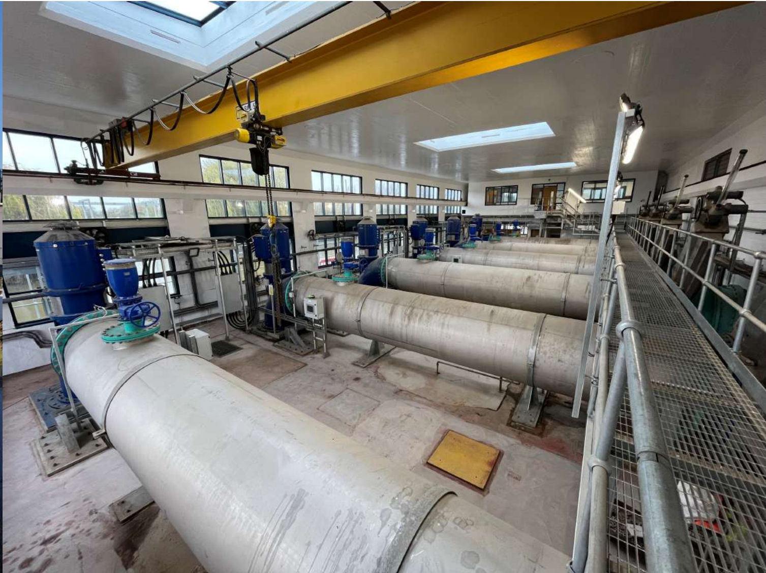
Keadby PS – 24m 3 /s capacity (6No 4m 3 /sec 330kW pumps)
