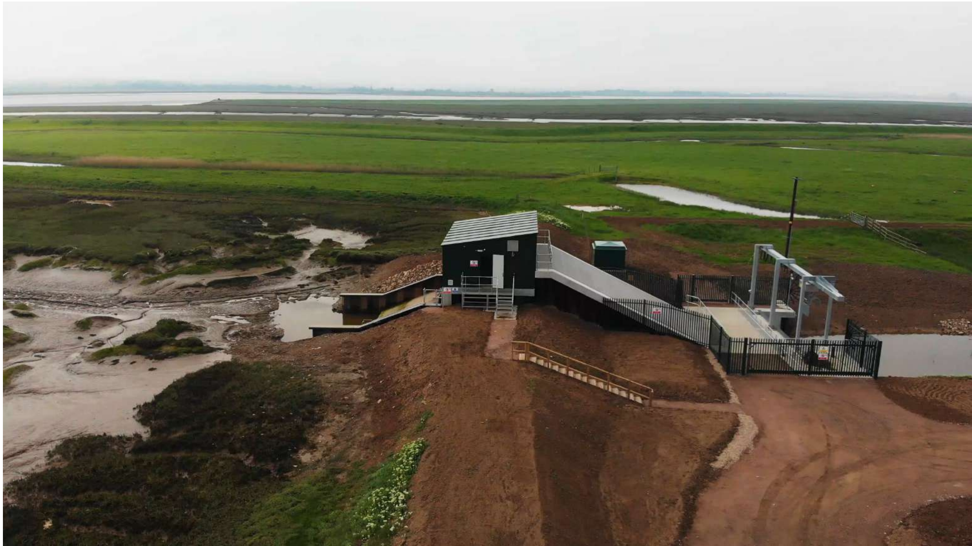
Bells PS – 3.5m 3 /s capacity (2No 1.75m 3 /sec 2m diameter screw pumps)
