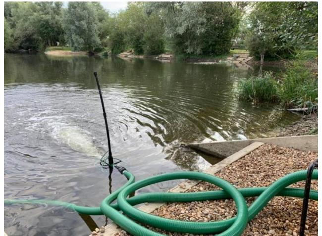
Check you have access to aeration equipment
