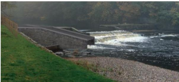
Low Mill weir on the River Wharfe at Addingham is a flow gauging station important for the forecasting of floods, and the management of water abstraction. We plan to install a new, efficient fish pass in 2017 (illustrated left).
