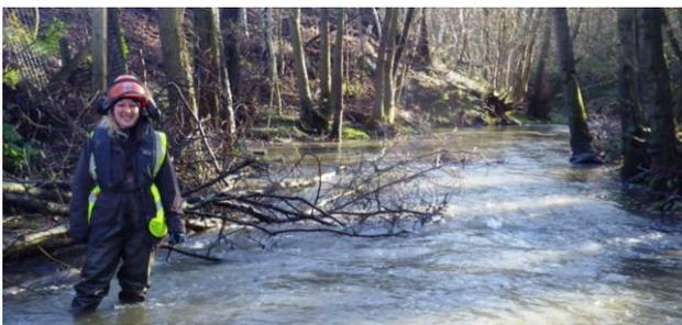
The River Stewardship Company has installed securely fastened woody debris into Barlow Brook, Chesterfield to provide cover for fish and increase the range of habitat available. We have also been helped by Chesterfield Borough Council and local landowners. Stock-proof fencing has been installed upstream to reduce sediment input.
