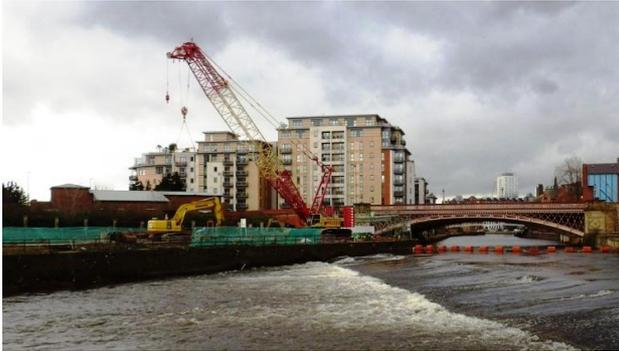
Work has begun on Knostrop and Crown Point weirs in Leeds as part of the Leeds Flood Alleviation Scheme. The weirs will be replaced with collapsible structures, to be lowered during floods. During normal flows the new weirs will be at the same height as the structures they replaced. Fish passes are being built to allow migration past these barriers.
