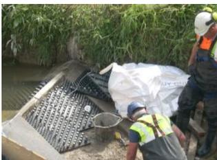
We are using studded tiles to help eels climb over some of our gauging weirs, such as on the River Kyle, Newton-on-Ouse.
