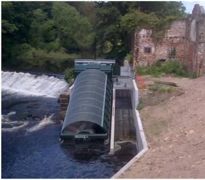
A new larinier fish pass has recently been installed at Goldsborough Mill on the River Nidd as a condition of the new hydropower scheme at the site.
