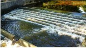
'Low cost baffle' fish passes have been built on our River Laver gauging weir, Ripon (left) and on Eshton Beck weir (right) where the pass was built in partnership with the Canal and Rivers Trust.
