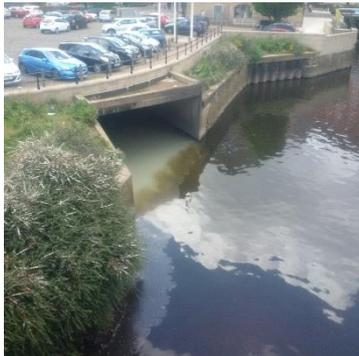
The Hol Beck in Leeds is a tributary of the River Aire, joining the main river in the centre of the city. Following reports of a white and oily substance, Environment Agency officers entered the culverted watercourse and located a likely discharge point. Dye testing was carried out to confirm the source. A discharge of contaminated site drainage was found and has now been stopped.
