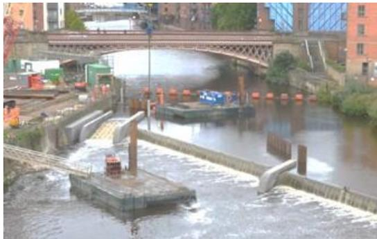
The fish passes on the River Aire at Crown Point and Knottingley are now both open. The Crown Point fish pass was built as part of the Leeds Flood Alleviation Scheme. The fish pass at Knottingley was a condition on the Environment Agency licence for the hydropower scheme on the weir.
