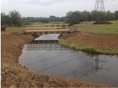
Working with Chesterfield Borough Council, we have re-connected over 0.5 km of historic meandering river channel to the Doe Lea at Norbriggs. The variety of depths and flows in the meanders provide a far better habitat for fish than the artificial straightened channel that used to bypass these features.
